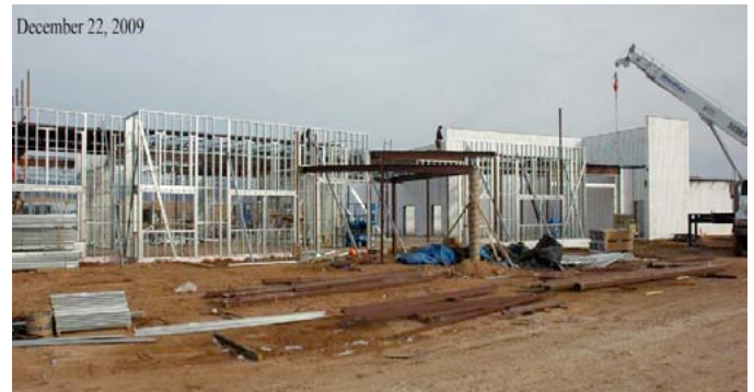
Underway – the entrance area of the new CNMA.
